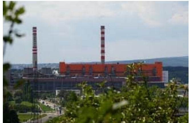
Heating plant Kosice, Slovakia
